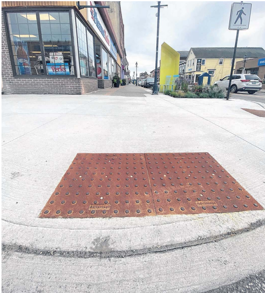
If you've seen these added to some areas in Yarmouth where sidewalks meet up with crosswalks they're to help alert people with mobility and visual issues that there is a transition happening from the sidewalk to the street. TINA COMEAU ■ TRI-COUNTY VANGUARD
